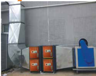
High Rise Building, Al Quoz
